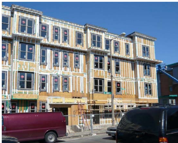
Figure 2.4. Dudley Village apartments under construction.
